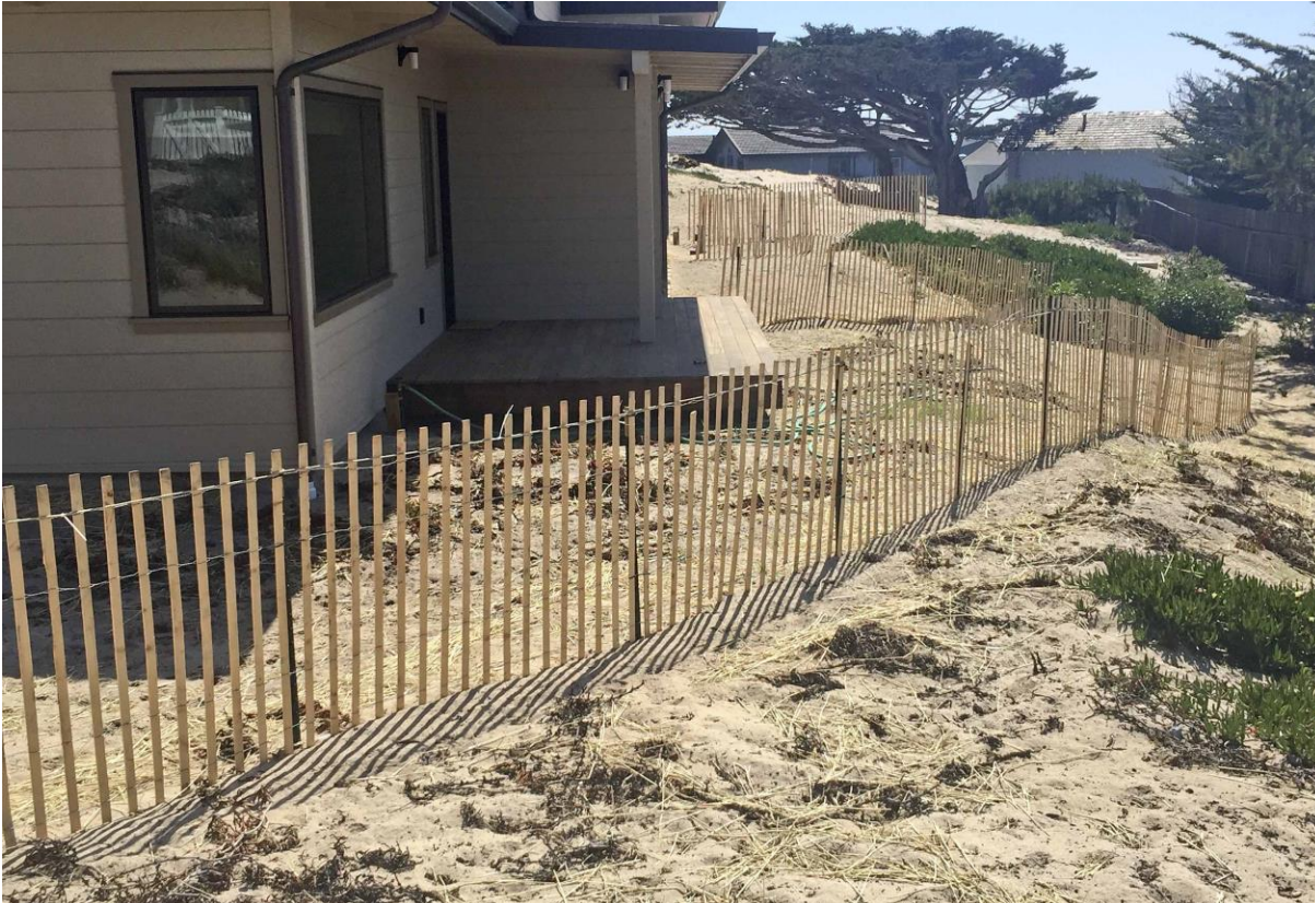
Photo 12. Example of temporary snow fence, used to control erosion caused by the wind.
